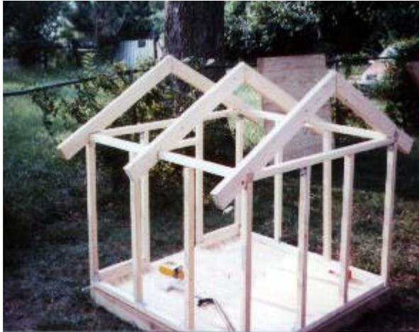
Fastening roof joists to frame. The 24 inch spacing of joists is nowadays bad juju in residential construction, but this is after all, a dog house with sixteen square feet of living area and a load of less than 100 pounds. I do not recommend going over the 24 inch spacing (take heed Irish Wolfhound aficionados).
