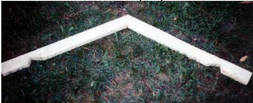
Roof "V" joist. Consists of 2x4 lumber with notches cut so that this form can rest atop the side walls of the structure. A tape measure revealed the notch corners to be exactly 48 inches apart, a perfect fit! Note that the apex of the inverted "V" was accomplished by careful "toe nailing" of the boards using at least six nails.
