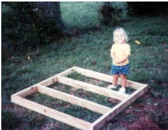
Floor Structure. Structure is a 48 inch square constructed of 2x4 pressure treated wood with joists at sixteen inch intervals. The lovely blonde model is about 34 inches tall.
