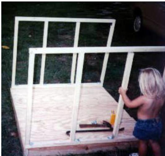
Side walls being attached to floor structure. Structure is constructed of 2x2 lumber with studs at sixteen inch intervals. Decking of floor is half-inch plywood. No children were harmed in the construction of this dog house.
