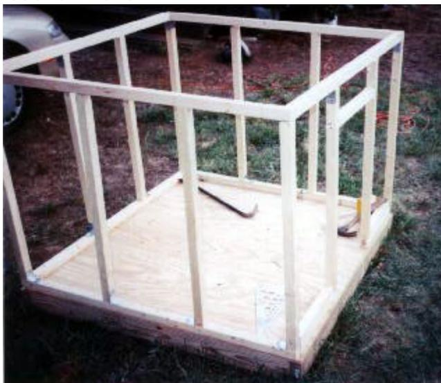
The total assembly of walls and floor. Note the use of "L" brackets at the corners for greater stability. If you are doing the job right at this point, the structure will become less flimsy as you attach one section to another.
