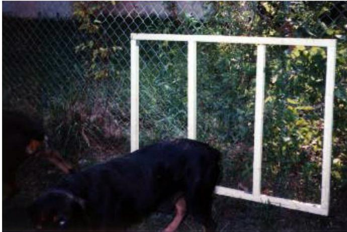
Side Wall Structure. Structure is a 48 x 36 inch rectangle constructed of 2x2 lumber with studs at sixteen inch intervals. As a bonus, you also see Mavis, a genuine blue-eyed Rottweiler, and the buttocks of Lana, her camera-shy mom.
