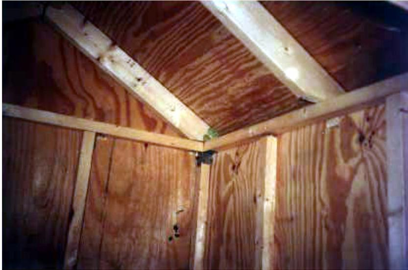
Interior shot of completed dog house. This picture reminds me of the slight gap that was left where the roof overhangs the side walls. I would be proud to tell you that it was a brilliant innovation designed from the very outset to provide adequate ventilation, but that would be a tissue of lies. It *is indeed* an innovation that provides ventilation, but it was the result of a jug head oversight. Thank you.
