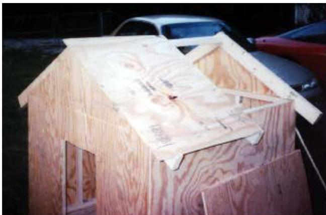
Roof decking being applied. Again with the plywood (three-eighths inch thickness). I would like to tell you that I used four sections of plywood because
